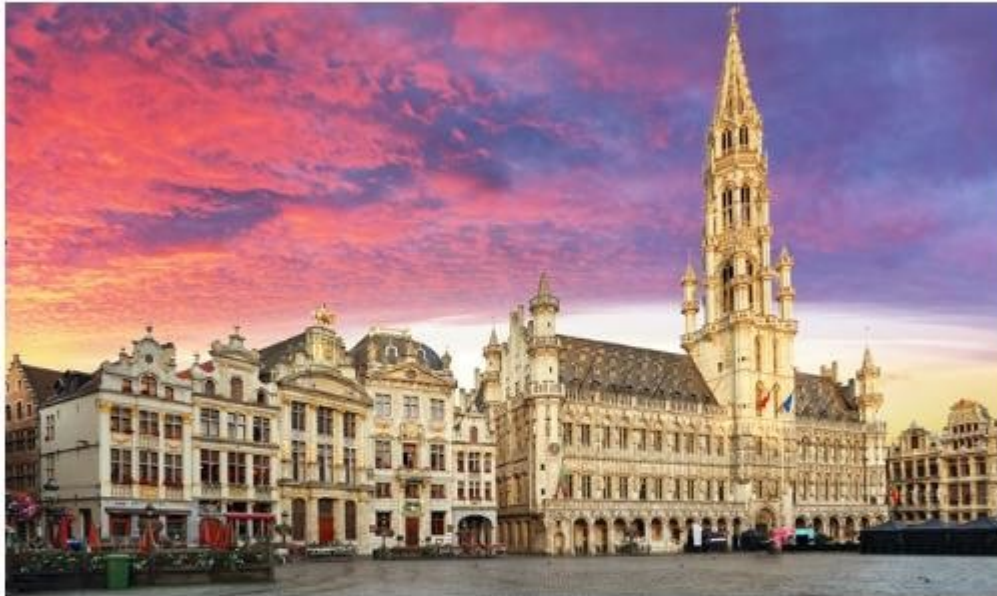
Grand Place in Brussels, Belgium
